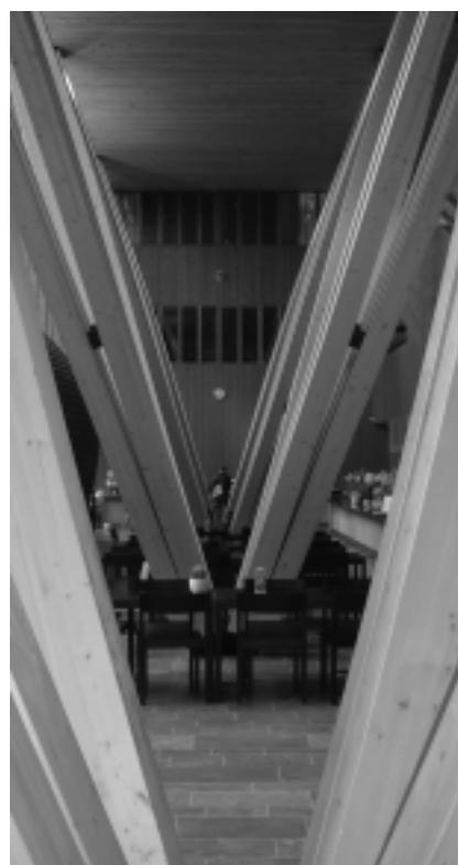
The Metla building in Joensuu is an example of the increasing interest in wood technology. 2000 m 3 of wood was used in its construction, in many innovative ways.
